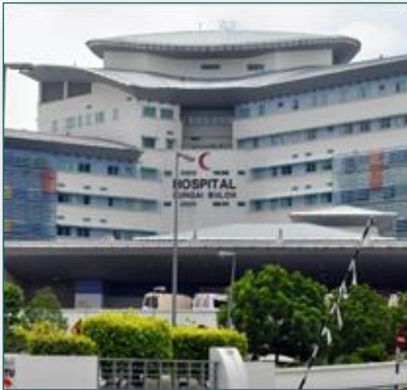
Sungai Buloh Hospital Malaysia Ebola room
